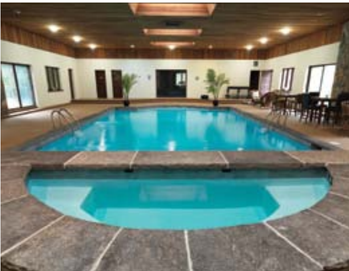
SILVER – Concrete Pool Renovation/Restoration
